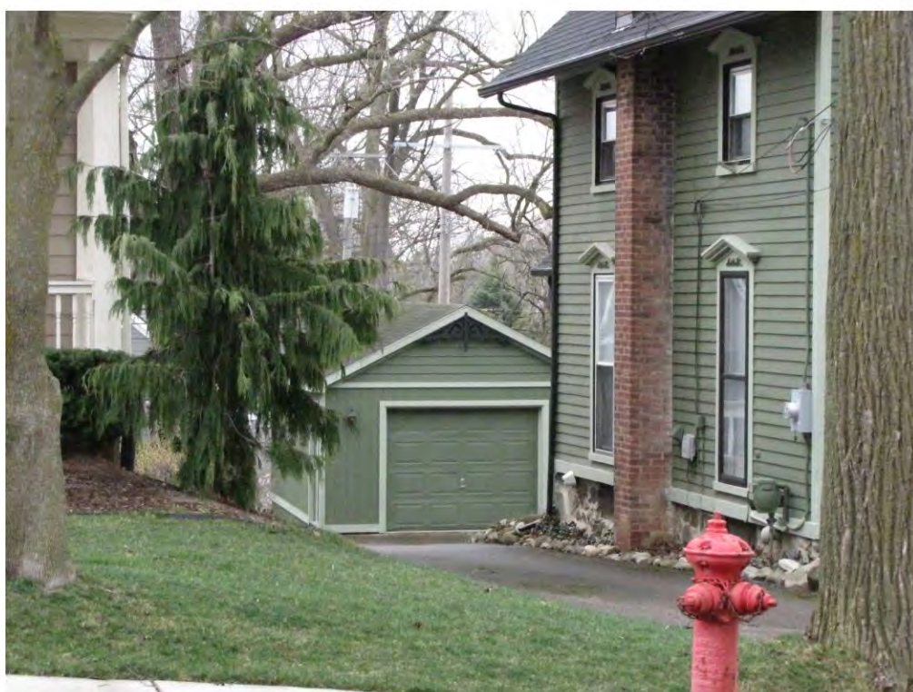
Rogers North 322, Garage_Looking East
