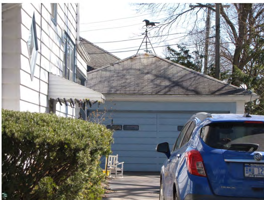
West 114, Garage_Looking East
