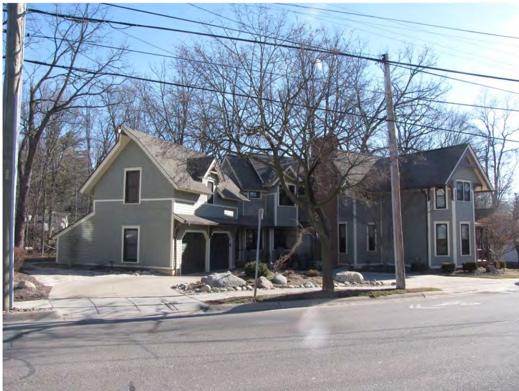
Randolph 402_Looking Northeast
