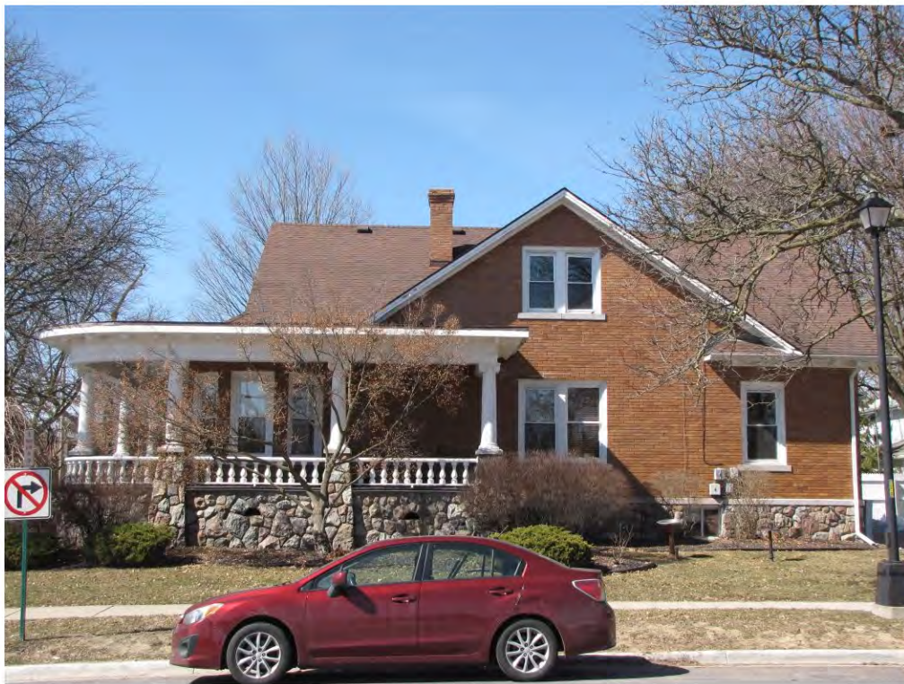
Main West 302_Looking West
