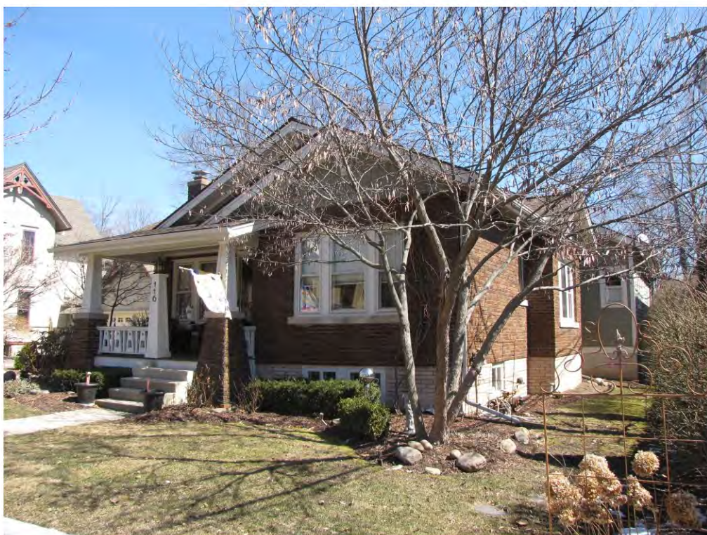
High 116_Looking Southwest
