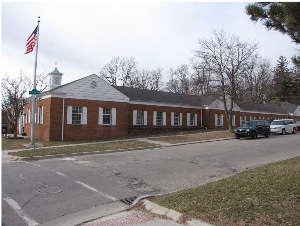
Wing South 200_Looking Southwest
