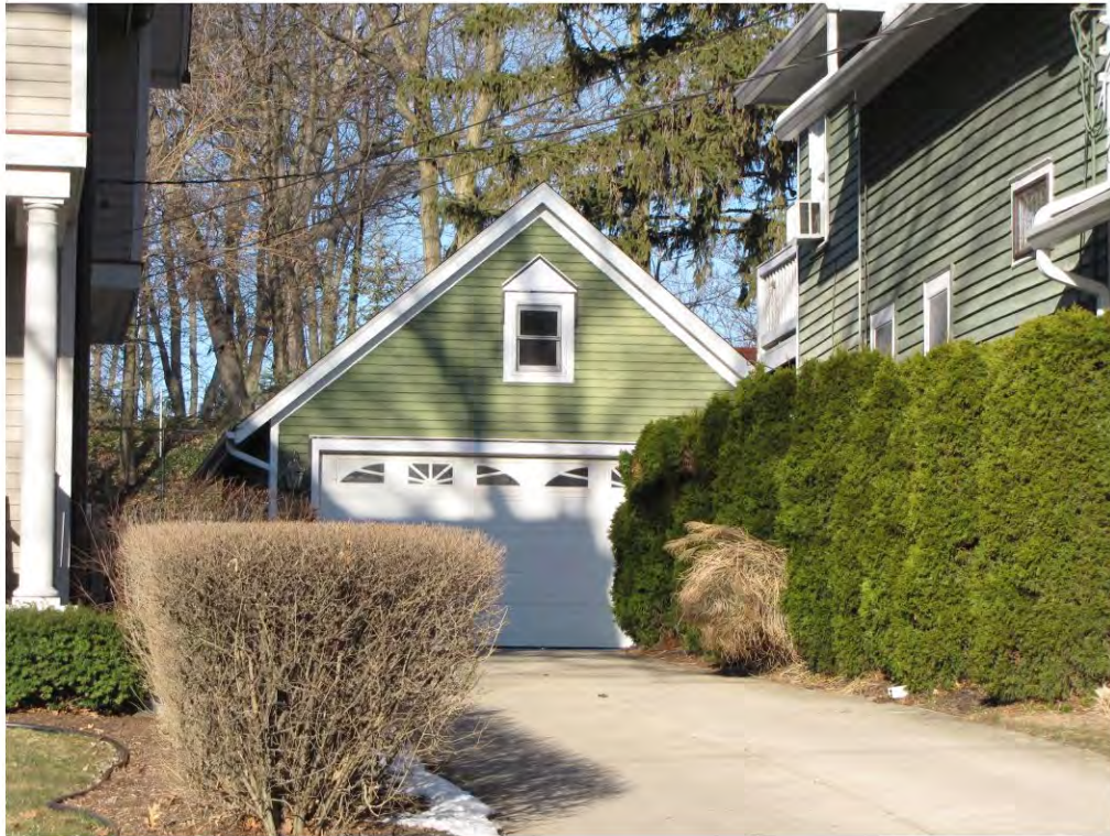
Rogers North 359, Garage_Looking West
