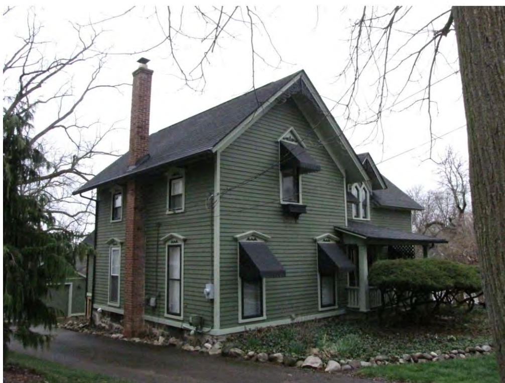
Rogers North 322_Looking Southeast
