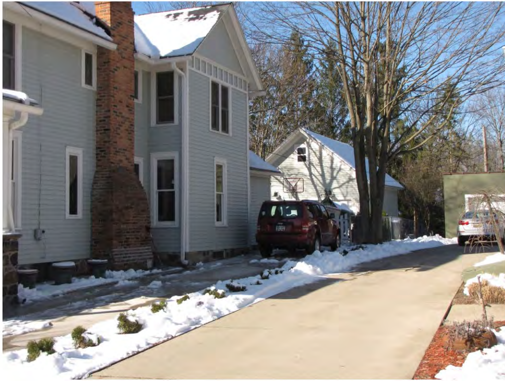
Rogers South 128, Garage_Looking West
